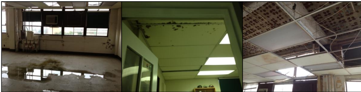
Figure 10: Pictures from Inside Building 669 (August 2012)
